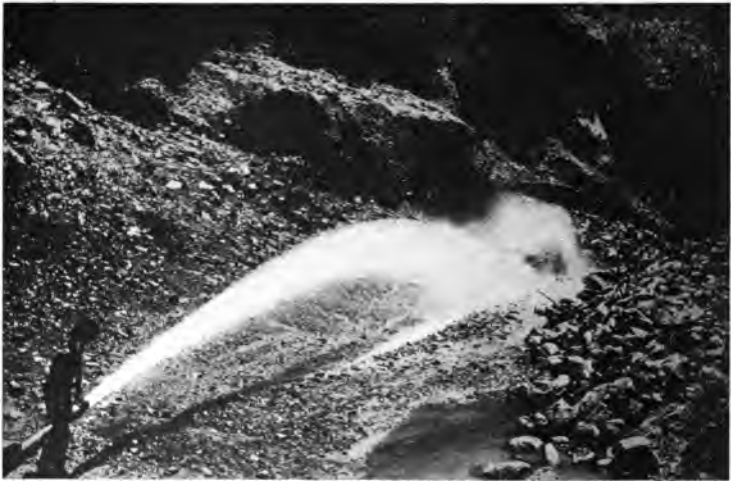
FIG. 100.—HYDRAULIC MINING ON THE KLAMATH RIVER, CALIFORNIA
